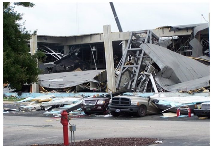
Graphical Representation of Building Damage Level 3
